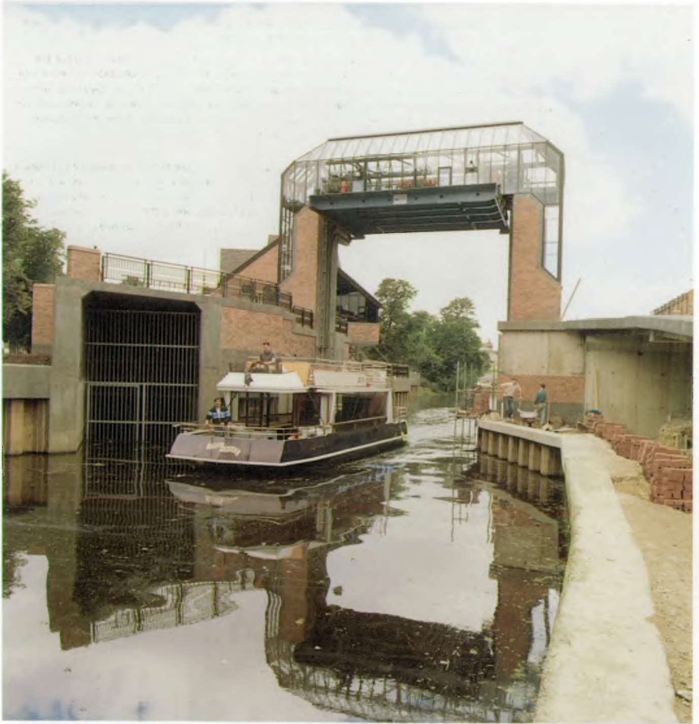
Discharge Culvert and Turn Over Gate
